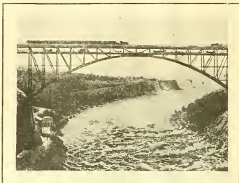
Single arch double track steel bridge over Niagara gorge on Grand Trunk Railroad.
